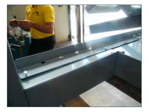
5) Place the filter on the appropriate section and fasten it with the supplied screws.
